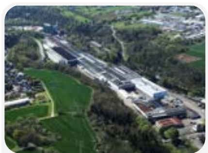
Location in Germany Production Facility, Neuwied (1500 m 2 )
